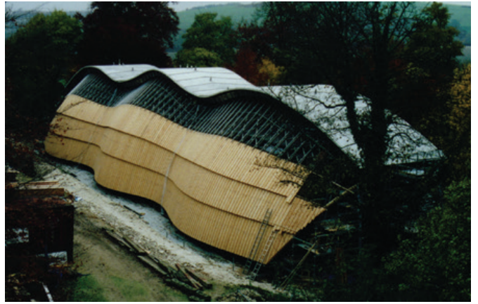
Above: The Gridshell was constructed as a flat carpet on a scaffolding about seven metres above the ground. The support was then taken away around the edges allowing the shape to drop towards an arched cross section. The sides were then pulled down and bolted to the edge beam, attached to a timber frame structure partially sunk into the ground.
