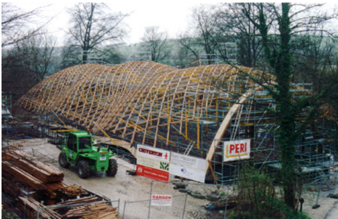
Above: The Gridshell was constructed as a flat carpet on a scaffolding about seven metres above the ground. The support was then taken away around the edges allowing the shape to drop towards an arched cross section. The sides were then pulled down and bolted to the edge beam, attached to a timber frame structure partially sunk into the ground.
