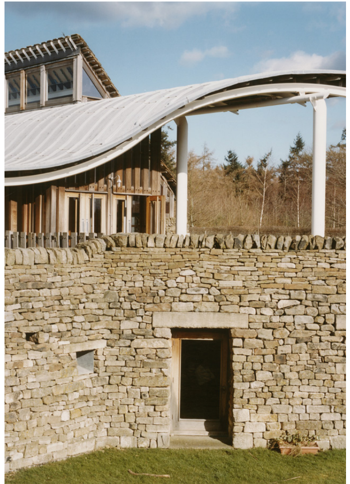
Curved lead roof with dry stone walls combine traditional materials with modern forms
