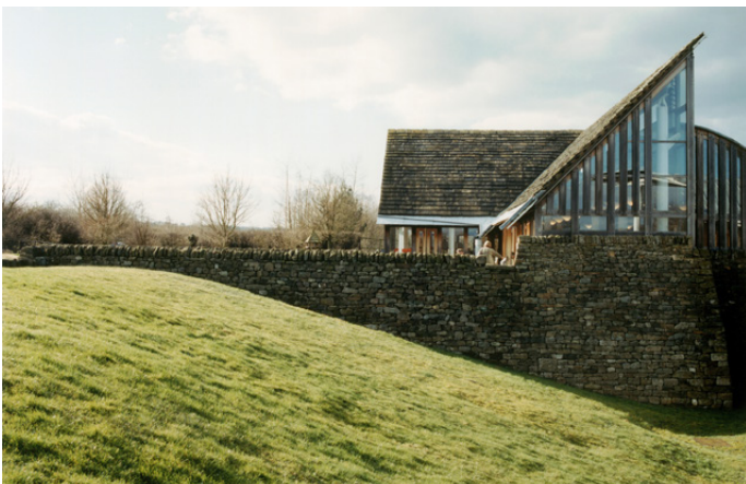
The visitor centre is stitched into the existing landscape and contributes a new one.
