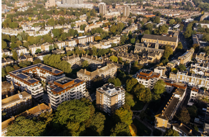
The Maitland Park Estate has been remodelled to better connect with its mature green landscape.
