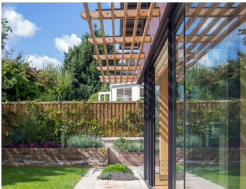
Above: Overhangs and bris soleil provide shade over large windows. Photo©Paul Raftery.
