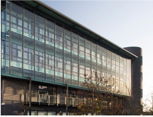
**Above:** Glazed panels on the double-facade open and close depending on the internal temperature of the building. *Photo©Simon Warren.*
