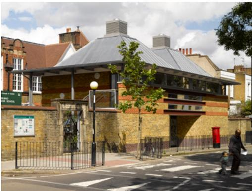
**Above:** The need to naturally ventilate the first floor hall has resulted in an exciting double roof form. *Photo©Edmund Sumner.*
